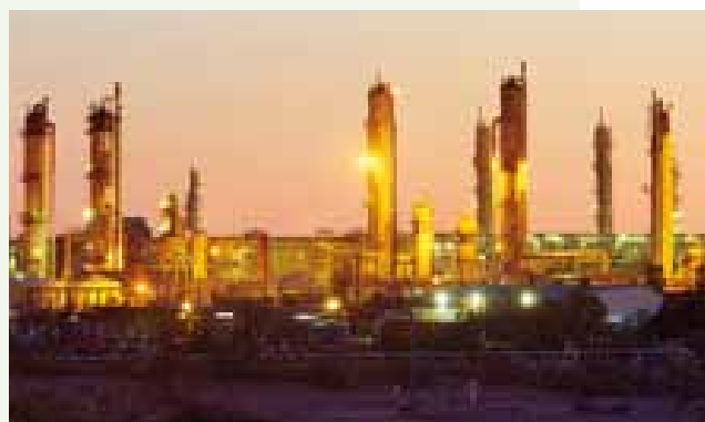
Moomba plant relocation and automation of the blow-down systems in the boilers will result in decreased water blow down volumes and associated energy savings.
